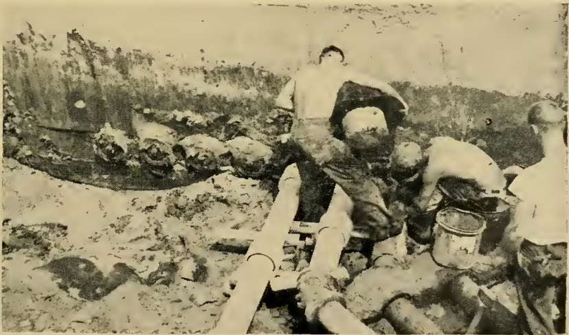
Sealing the joints in the piping between the pumping station and the settling tank.
