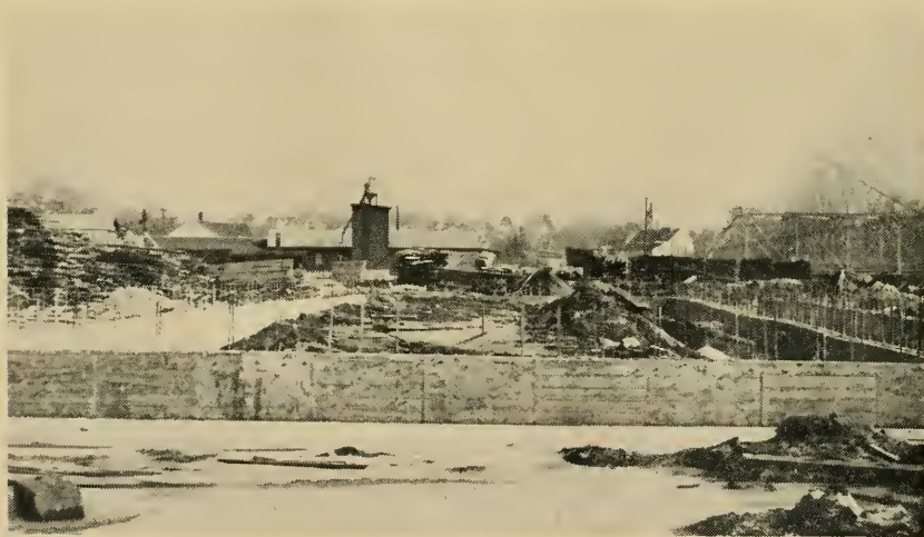
Laconia Sewage Disposal Plant, showing foundations of the Sludge Drying Beds. See page 52.
