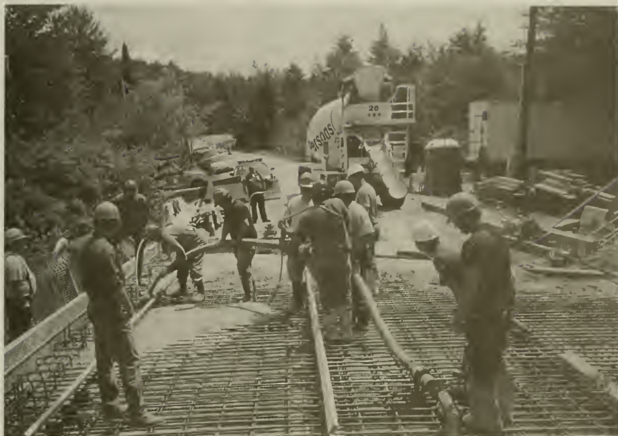
POURING CEMENT ON FRENCH ROAD BRIDGE
