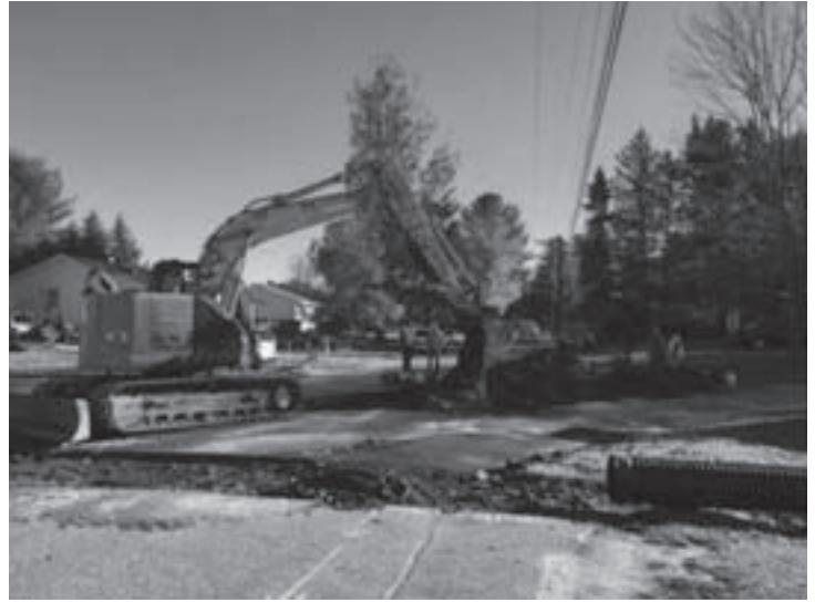
Removing and replacing old drainage structures on River Road
