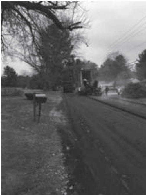
Repaving part of River Road
