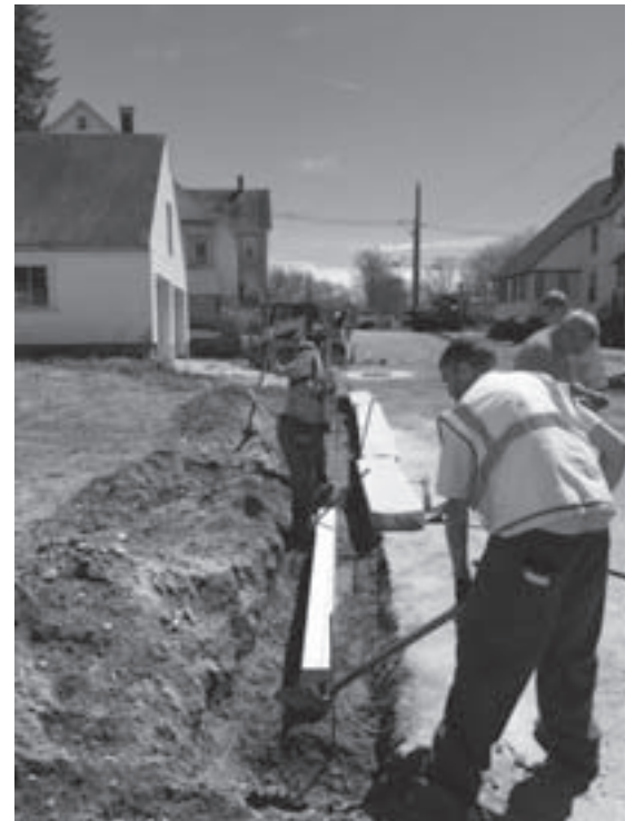
Installing a new curb on Reynolds Avenue
