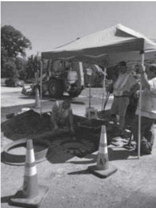
Raising a drainage manhole on Ferry Street
