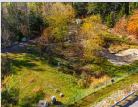
The University of New Hampshire Stormwater Center Field Site, adjacent the university’s West Edge Parking Lot. The site is designed to provide an apples to apples comparison of how stormwater treatment systems reduce pollution and manage the volume of runoff.
