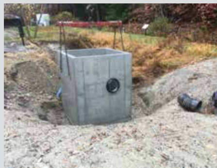
Three new manufactured systems were installed at the UNH Stormwater Center’s field site in fall of 2019.
