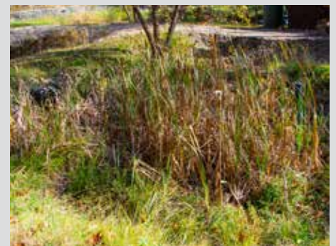
Un-maintained gravel wetland at the field site reflects the standard of practice and is an excellent opportunity for research to support operations and maintenance for this system.
