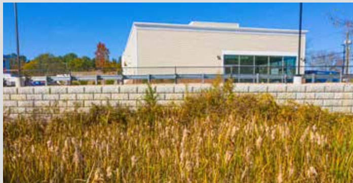
Filtration systems like this subsurface gravel wetland fit seamlessly into the landscape and improve water quality.
