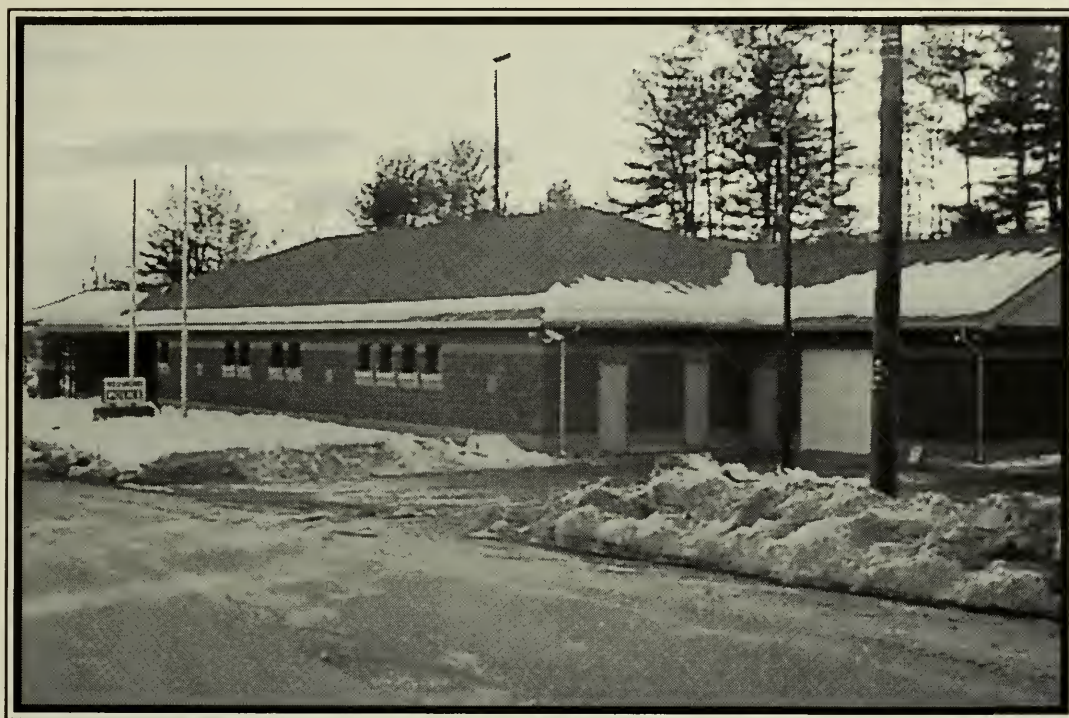
Hillsborough Police Station Built 1997
