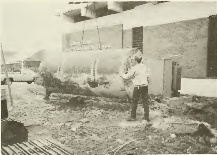
Employees complete removal of 8500 gallon and 2500 gallon underground fuel tanks.
