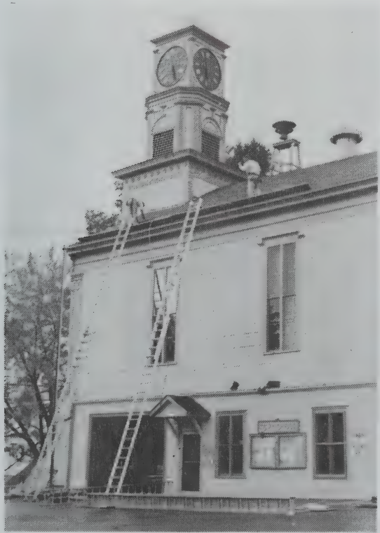
Town Roof Repairs
