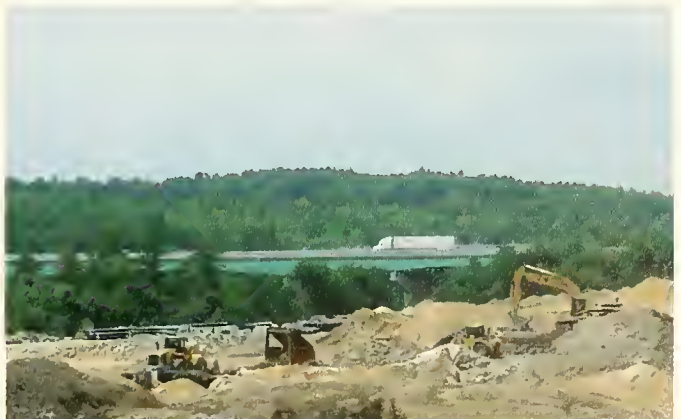
Hooksett Crossing -Home Depot Construction
