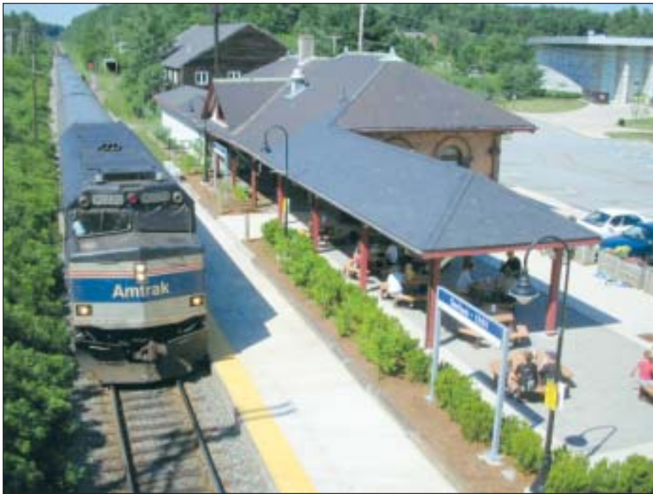
The Amtrak Downeaster Durham station was opened in 2001 and continues to increase its ridership and thereby provide an alternative to travel in single-occupancy vehicles. During March 2004, approximately 1,300 individuals departed and arrived at the UNH station.
