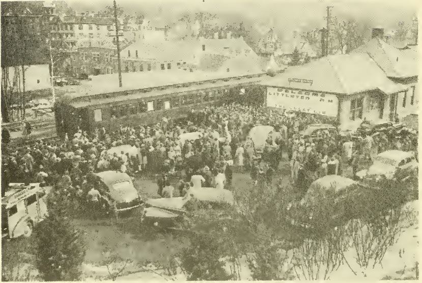
Awaiting Bette's arrival at the Littleton Railroad Station.
