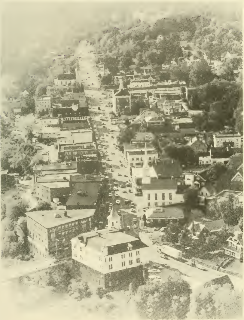
This aerial shot of Littleton, taken from the Town Hall end of Main Street, depicts Littleton's active downtown district which is regionally recognized as a major shopping area in the White Mountains.
