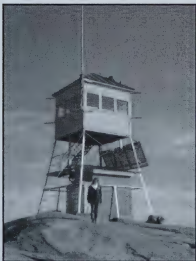
The tower as it stands today
