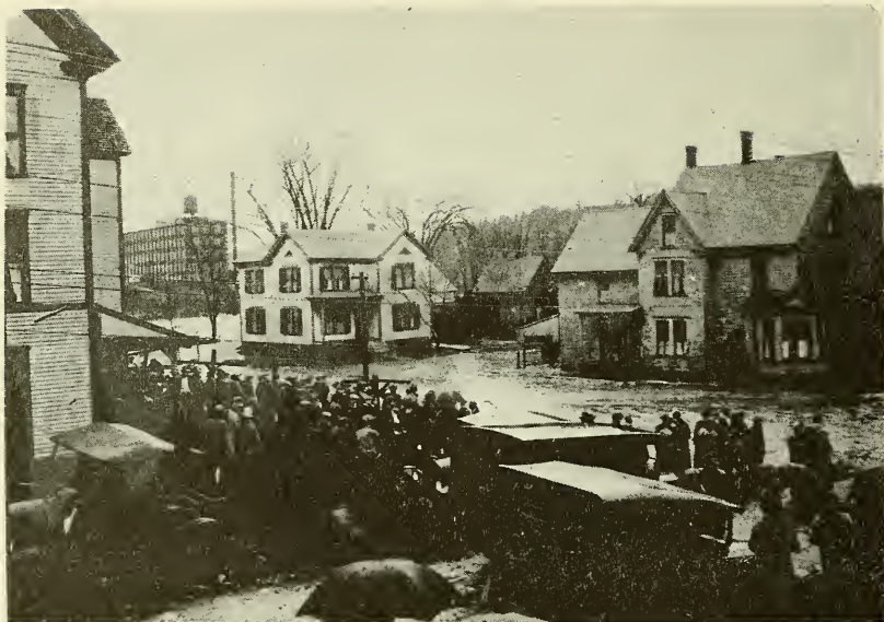
Flood On Lafayette Avenue — Devastating flood of 1927 as seen on Lafayette Avenue; Sears Roebuck factory is seen in the rear.
