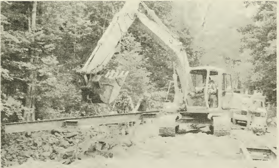
Ball Park bridge drops in place.
