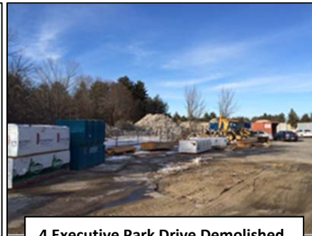
4 Executive Park Drive Demolished
