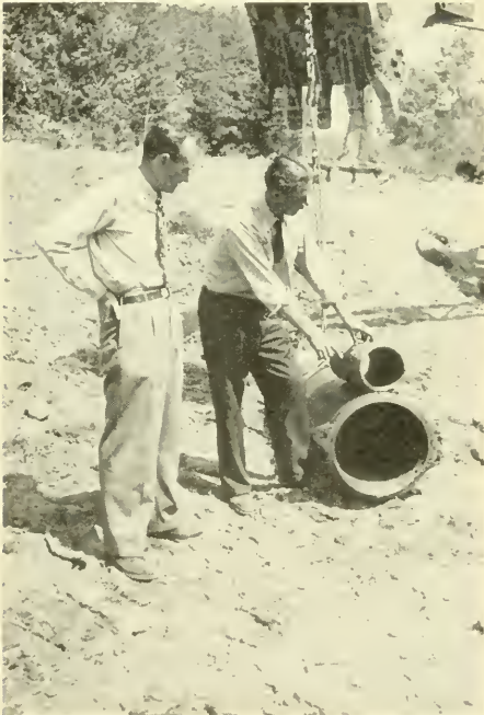
Superintendent of Public Works compares the old, undersized mains with the pipe which now brings water to Keene from Roxbury.
