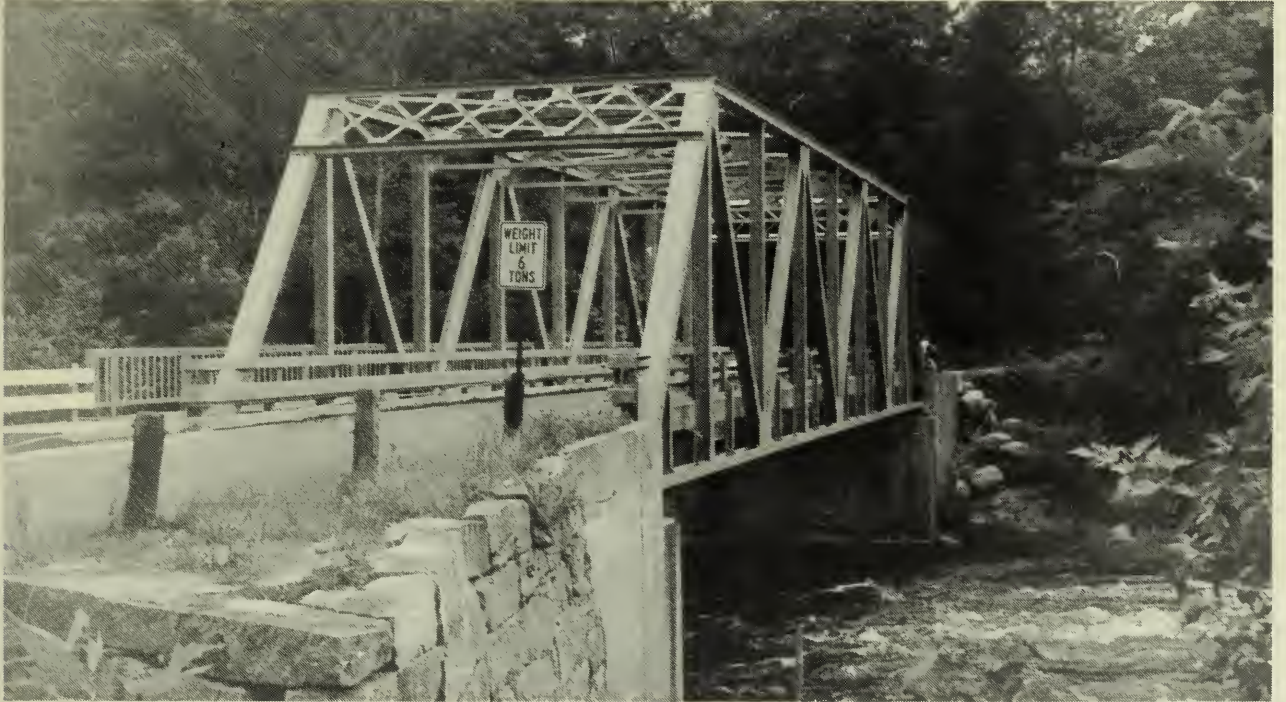
July 1988 Refurbished Bridge
