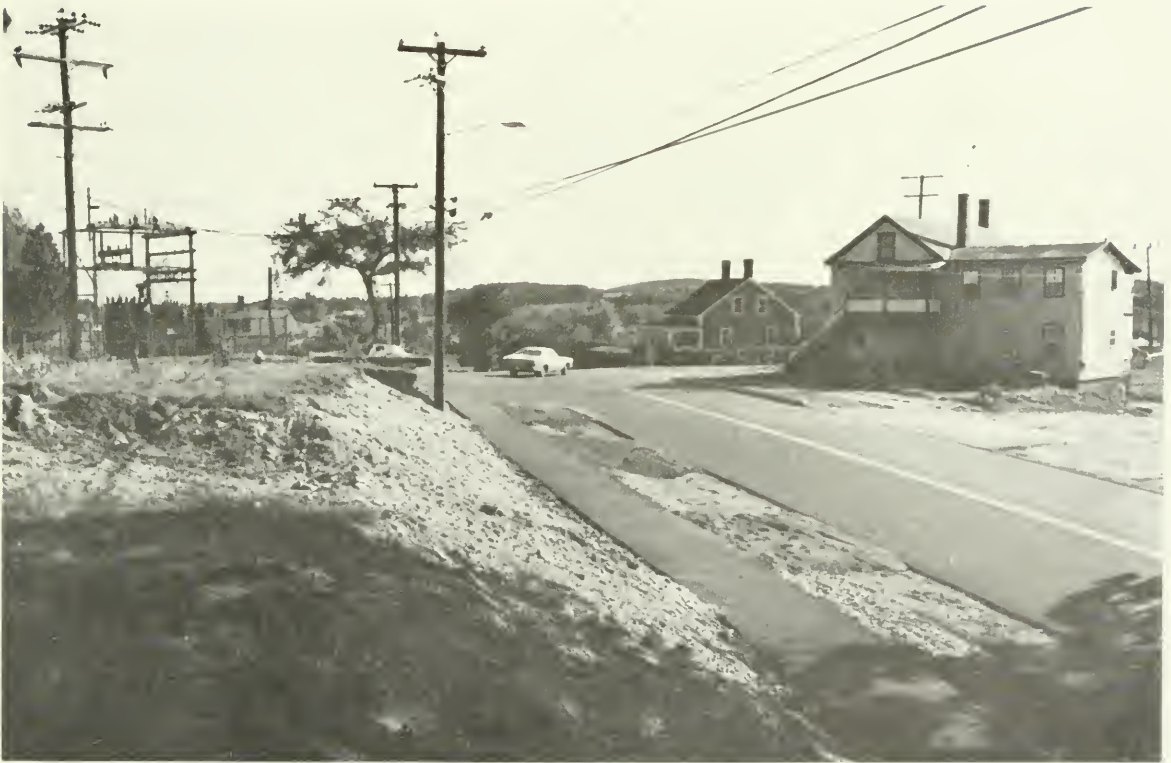
Green Street Reconstruction
