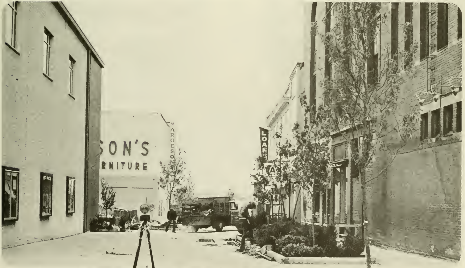
The new Vaughan Street Mall nearing completion.
