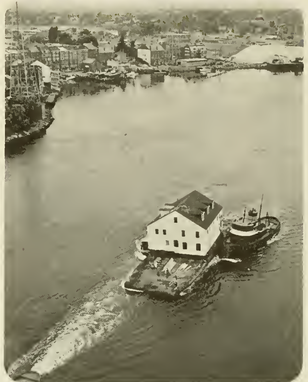
The Joshua Wentworth House being moved from the Vaughan Street project to Strawbery Banke.
