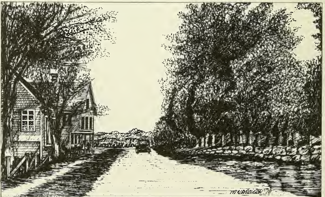
CORNER STORE GARRISON ST. NOW KINGSTON RD.
