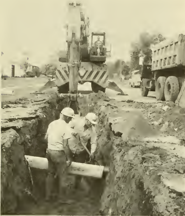
Maple Haven Sewer Project
