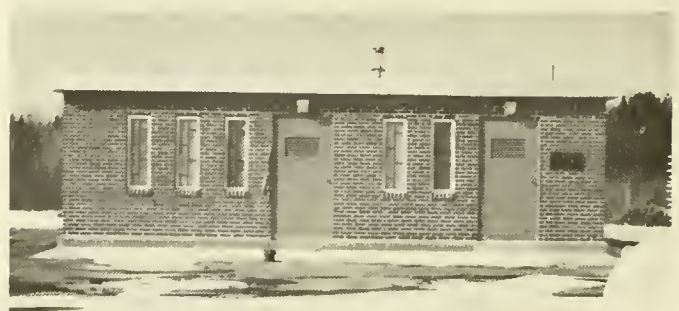
Rye Line Pumping Station
