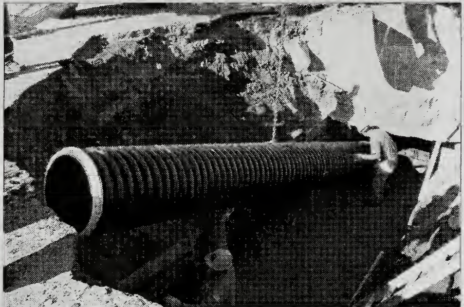
Canal Reconstruction under Depot Square Parking Lot
