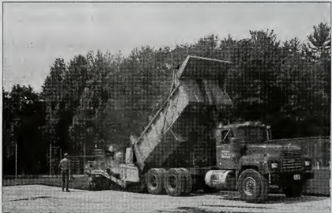
Paving of Adams Playground Tennis Court
