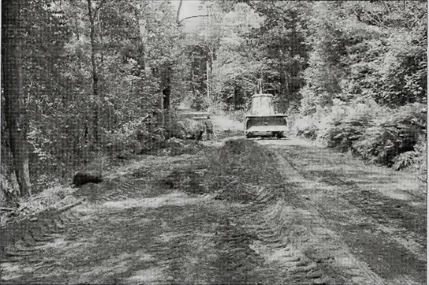
Construction of Four Winds Farm Road Photo by Ed Betz
