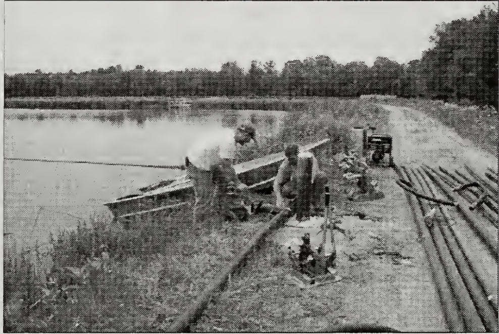
Installing lagoon aeration at the wastewater facility
