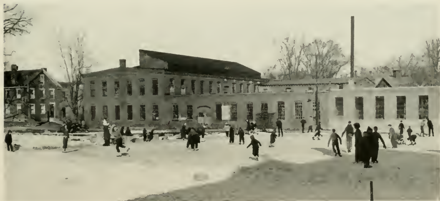
The new skating rink on the former A. E. Fish Company property brought joy to hundreds of youngsters.
