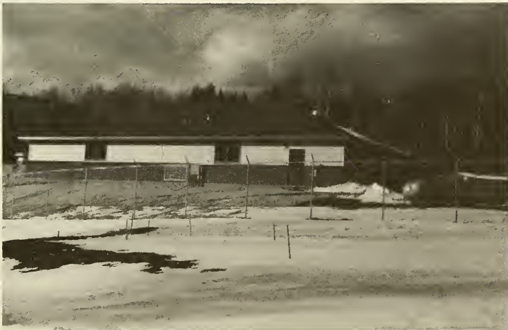
New Water Filtration Plant located on Jintown Road.
