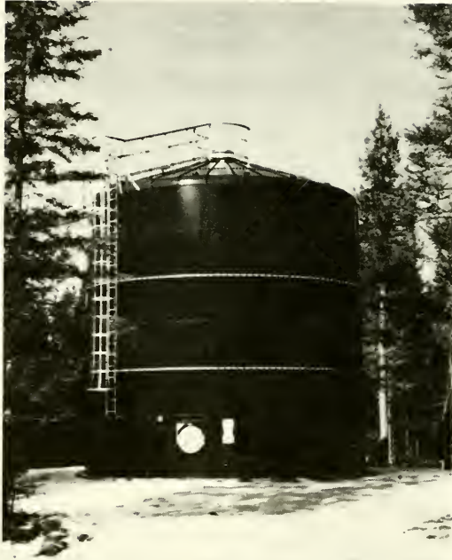
Water Storage Tank at Little River Road
