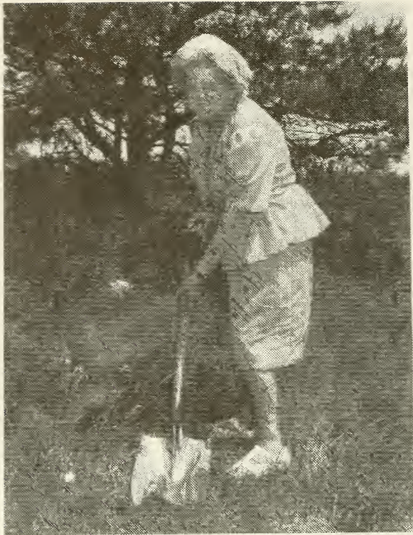
Ground is broken by committee member Lydia M. Gould . . .
