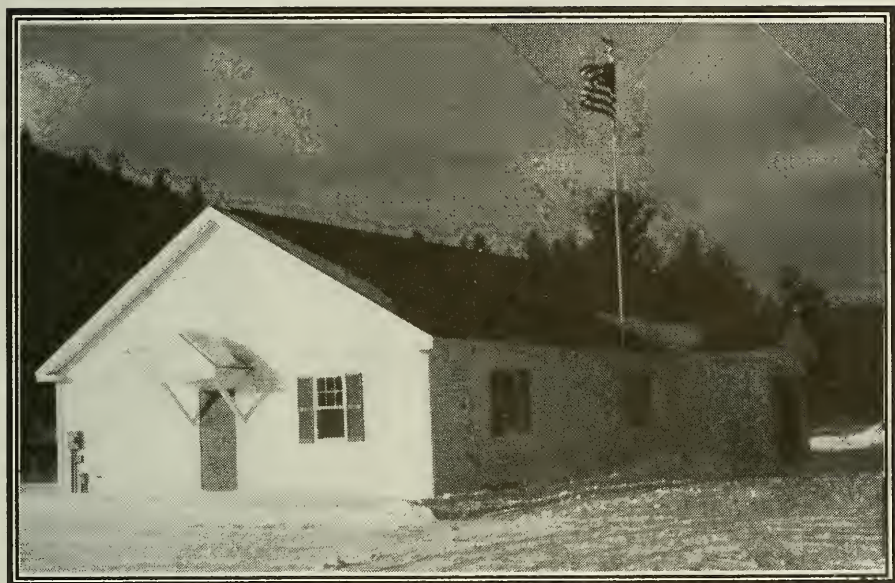
RUMNEY TOWN OFFICE BUILDING Constructed September 1991-January 1991
