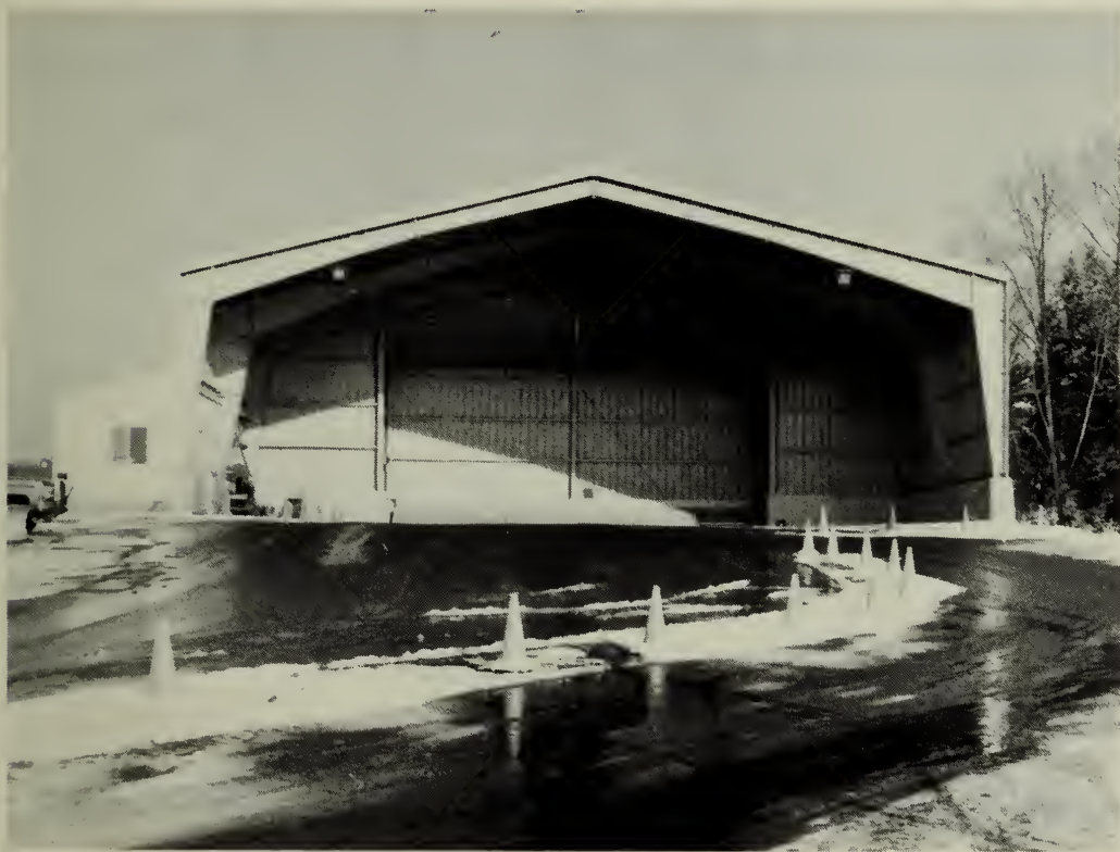
HILLSBOROUGH SOLID WASTE TRANSFER STATION
