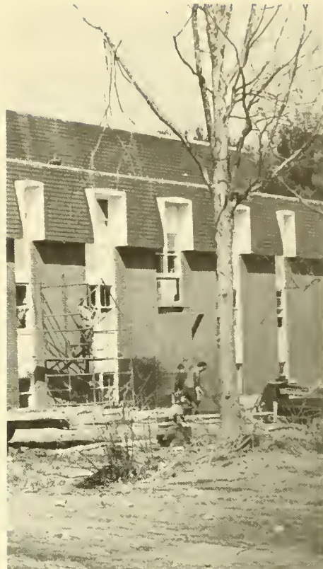
New apartment construction means extended water, sewage lines.
