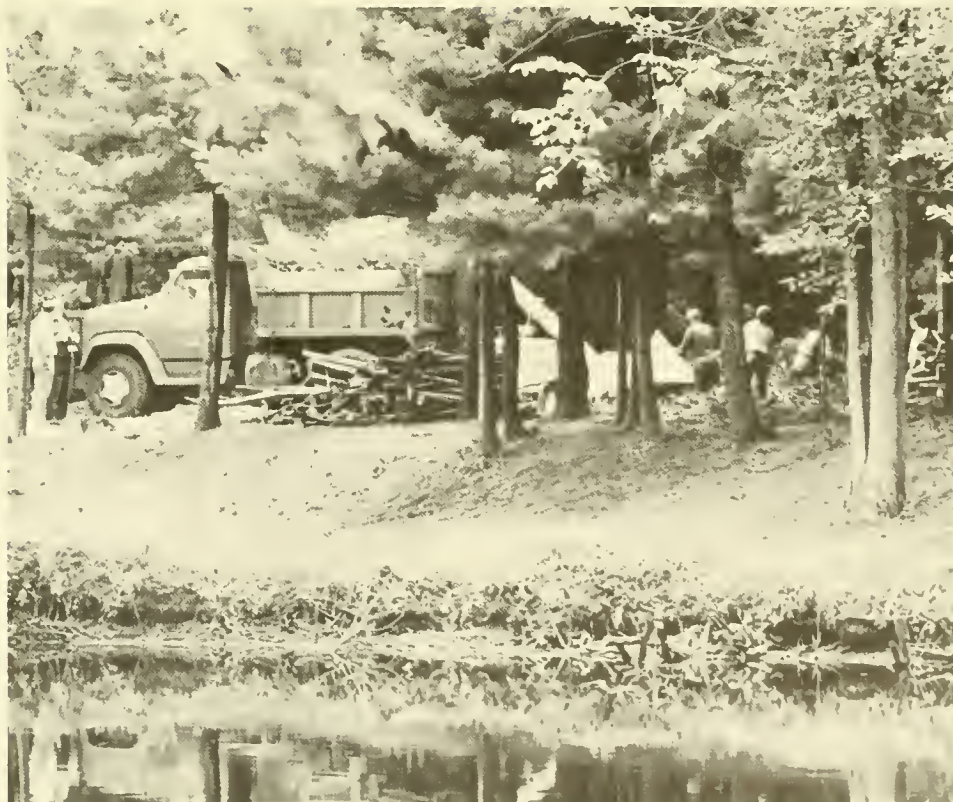
Public Works crews assist on park development project.
