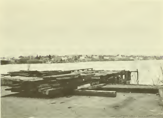
Rehabilitation of Prescott Park Wharf.
