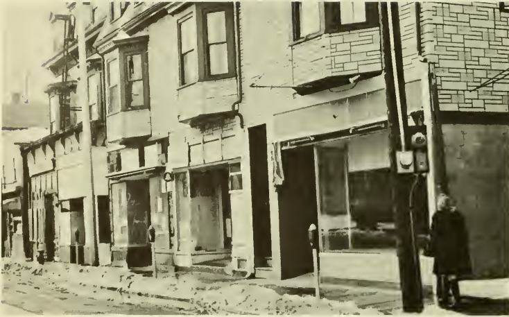
Vaughn Street Urban Renewal Project, Congress St.
