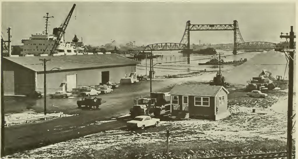
New Hampshire State Port Authority Terminal and Memorial Bridge.
