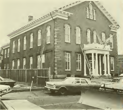
Complete window renovation in City Hall.
