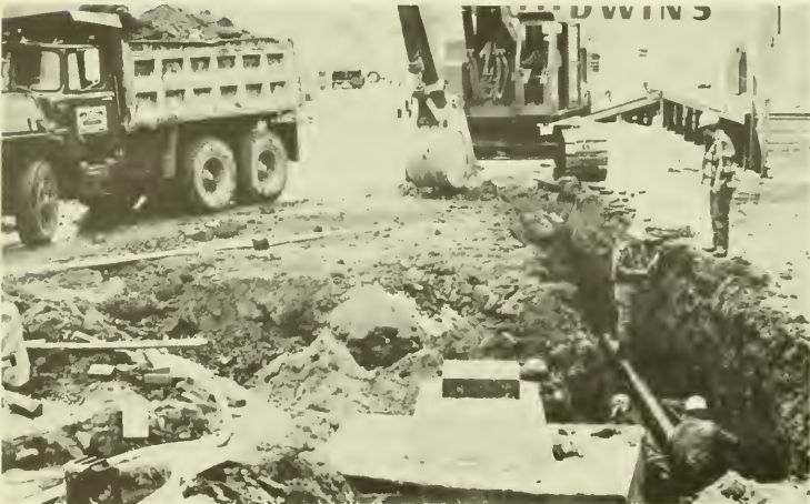
Laying of utilities within the Urban Renewal Project.
