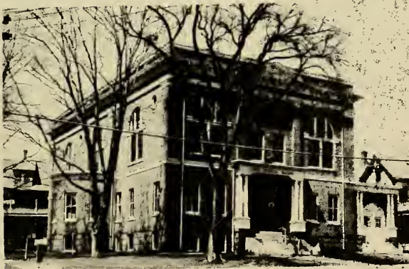
Adams Memorial Building
