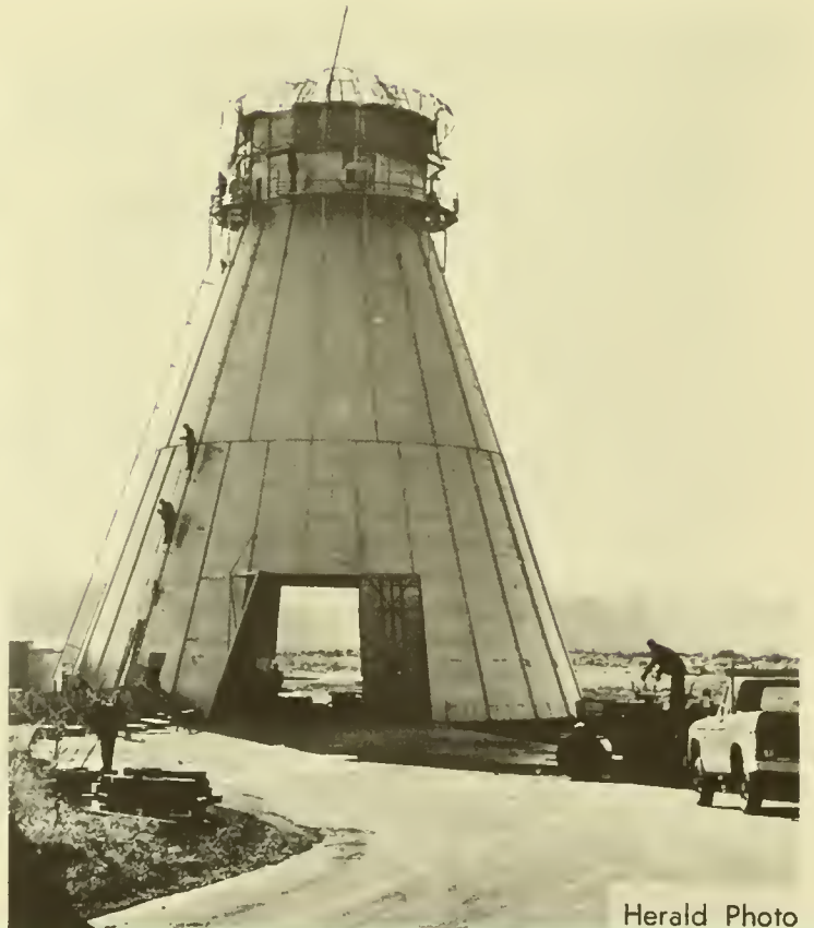
Construction of Cone-Type Incinerator Jones Avenue Dump Area
