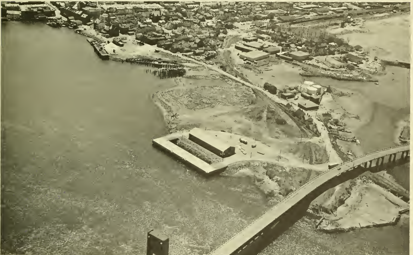
New Hampshire State Port Authority Wharf
