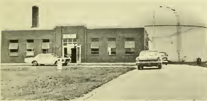
Water Department Bean Hill Control Station
