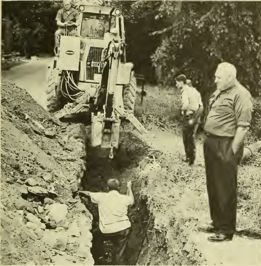
Water Department Banfield Road - 10 in. main extension
