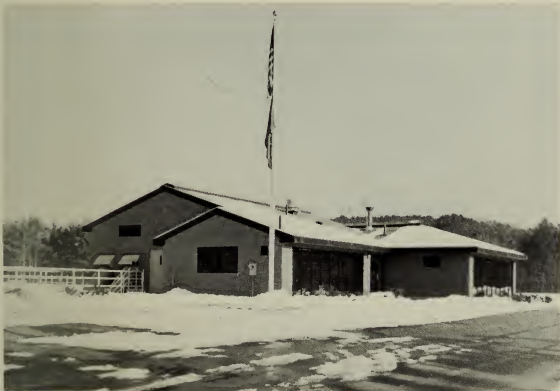
HILLSBOROUGH WASTEWATER TREATMENT FACILITY
