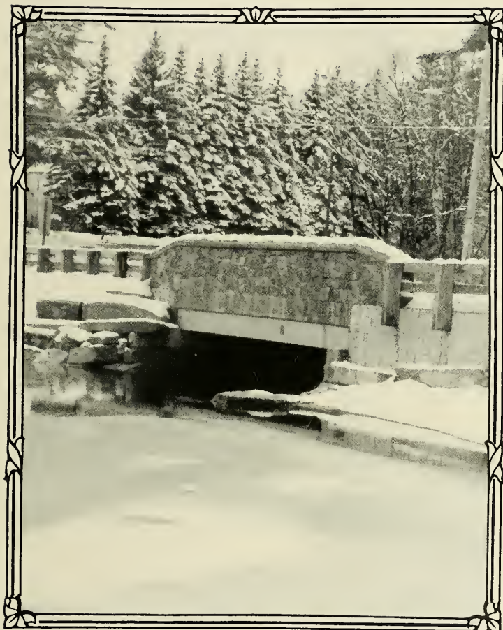
Mill Street Bridge, Center Conway, New Hampshire Reconstructed 1994
