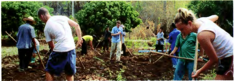
UNH engineering students help dig a leach field in Santisuk, Thailand.
