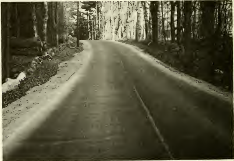
Allard Hill Road reconstruction
