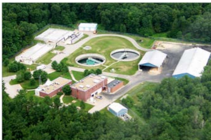
Figure 16. Aerial photo of Dover's WWTP.
