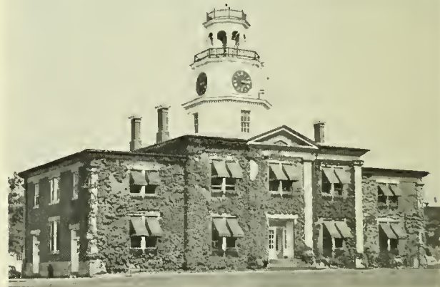
Administration Building, Portsmouth Naval Shipyard. Contains first clock in the United States to strike "ship's bells." Invented in 1894 by Alvah Frost of Kittery, a civilian worker.
