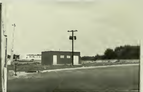
Completed Sewerage Pump House
