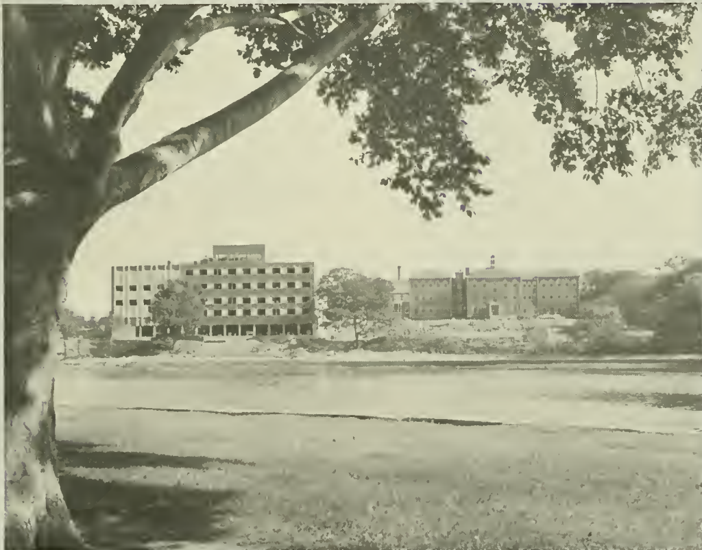
New Portsmouth Hospital Construction — South Mill Pond Shore and Junkins Avenue.
