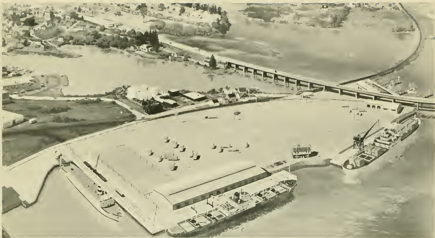
Artist's Rendition of New Marine Terminal on Nobles Island — New Hampshire State Port Authority.
