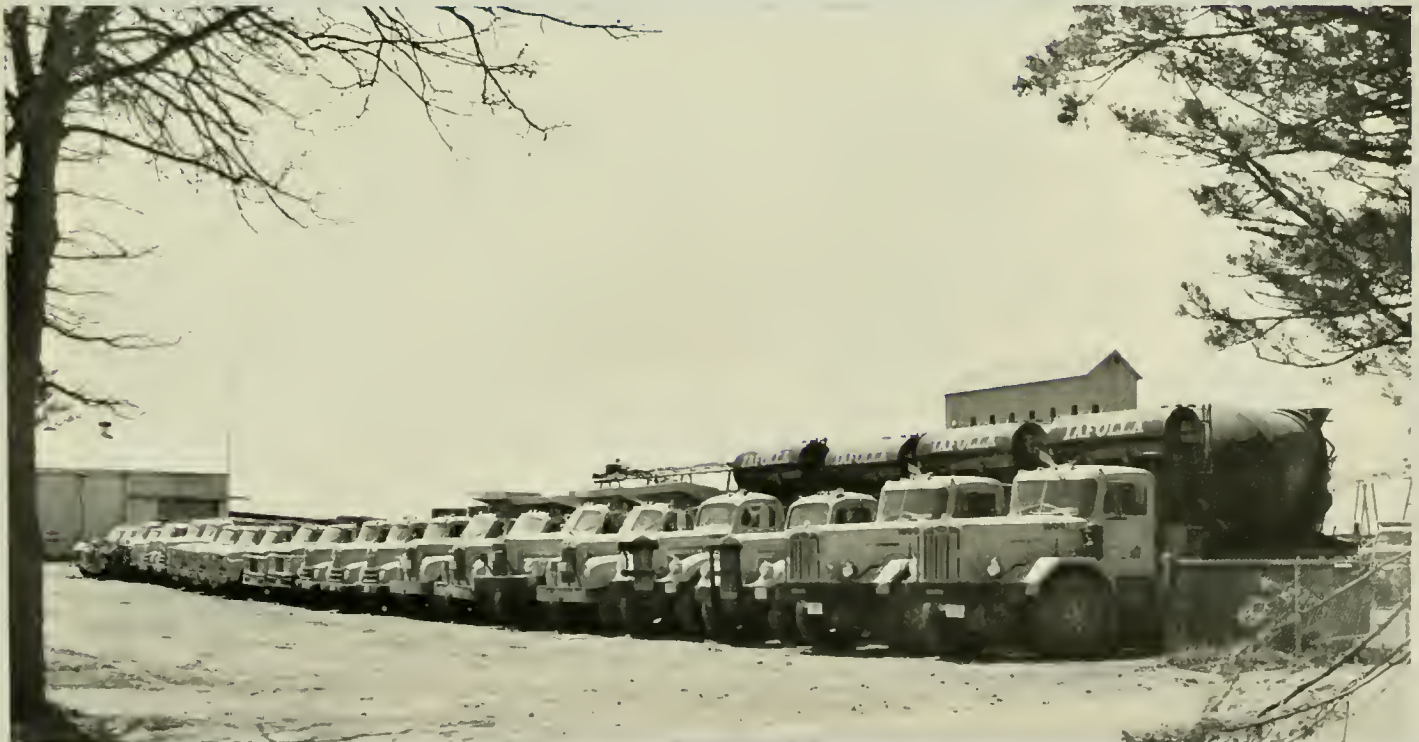
Delivery Equipment — Peverly Hill Road — Iafolla Construction Company.
