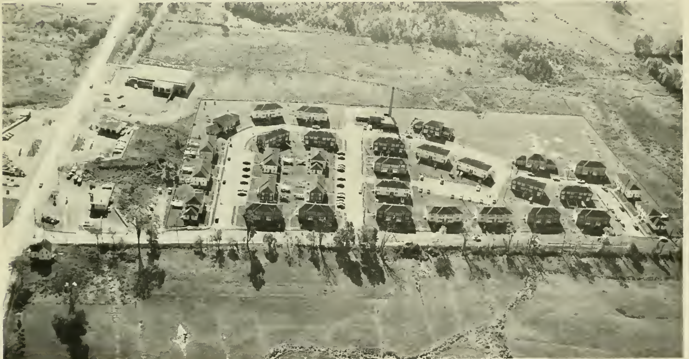
Public Housing — 124-Unit Project Area — PHA — Gosling Road
