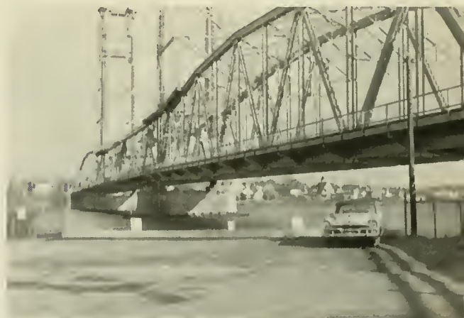
New Snow Dumping Area
