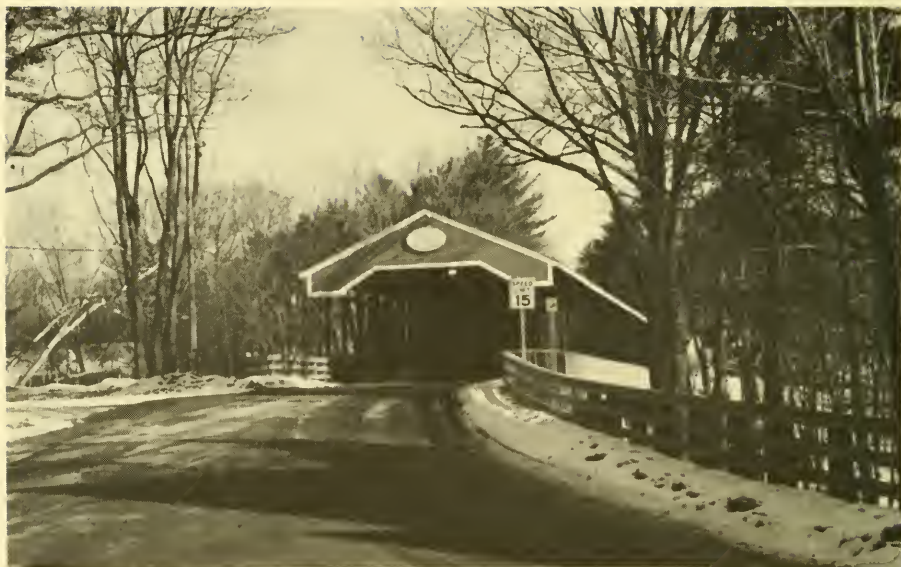
SACO RIVER COVERED BRIDGE Reconstruction completed May, 1989
