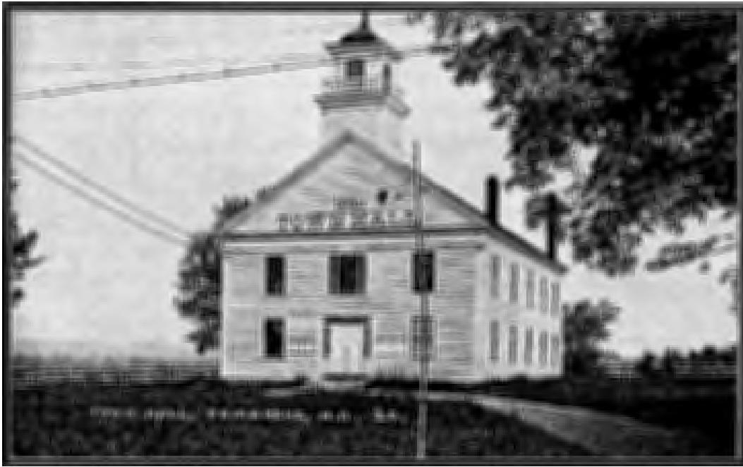
Original Pembroke Town Hall
