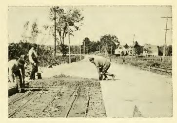
Reinforcing the Strength of the Road with Ribs of Steel.
