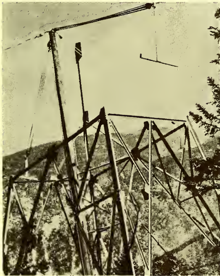
Gin pole being used in erecting one of the intermediate towers and Mountain Station.
