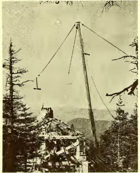
Gin pole being used in erecting one of the intermediate towers and Mountain Station.
