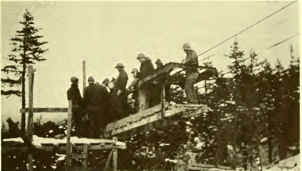
The freight tram car with a load of construction workers near the Mountain Station. Communications to the operator in the valley was with a telephone magneto and an insulated metal prod. The trick was to reach out far enough with the prod to contact a telephone wire while spinning the magneto crank. Photo by D. Champagne.
