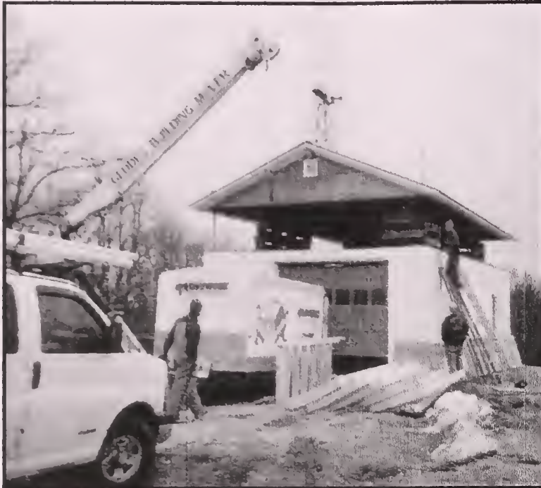
Above Left: Dave Hewey (on ladder) works to raise the roof at the Sugar Hill Fire Station to enable housing of larger equipment.
