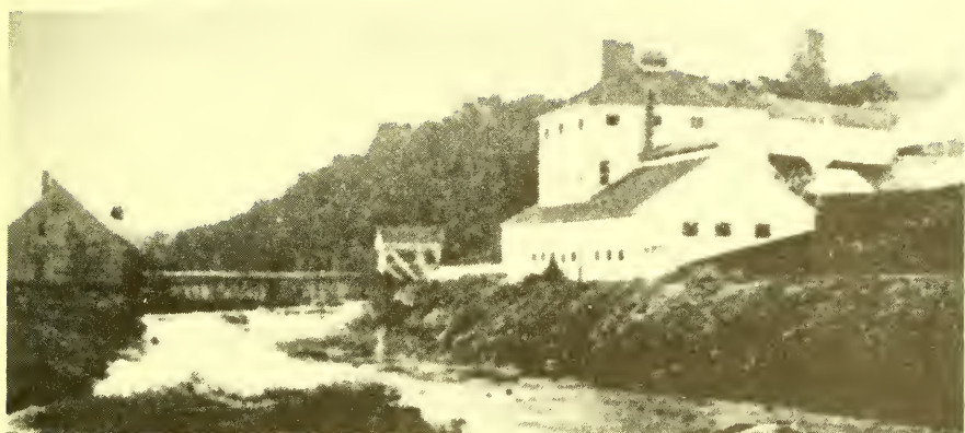
An 1875 picture of the New Hampshire Iron Works (1805 to the Civil War). The present stone stack, about all that remains, was contained within the buildings shown. The dam above the mill provided power for a grist and lumber mill on the left bank.
