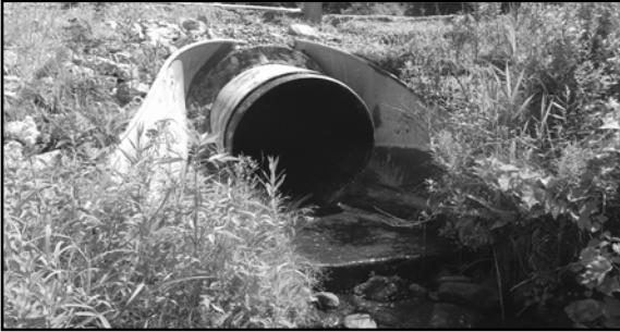
Photograph looking at the discharge end of the new 36” diameter HDPE culvert pipe (black round pipe) that was slip-lined through the existing 42” diameter failed corrugated metal pipe. The annular space between the two pipes is filled with a high strength grout upon completion of the slip-lining process.
