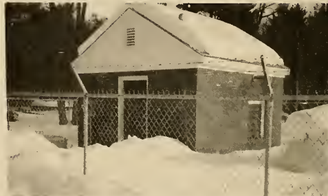
Lift Station – Haigh Ave.
