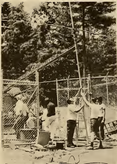
Erecting Antennas for the Emergency Drill held in June.
