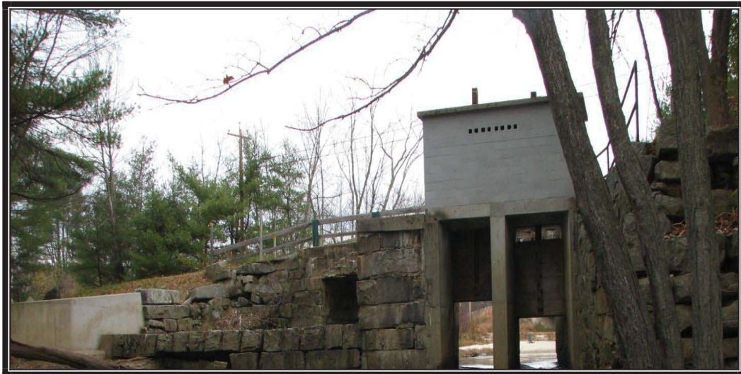
Buck Street Dam East
