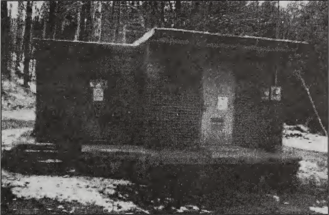
Old Chlorine House (Before Upgrade)
