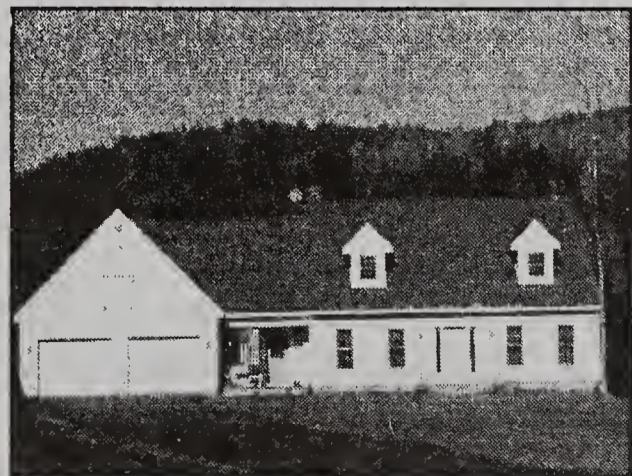
New Construction - Burnham Julie Collins Photo
