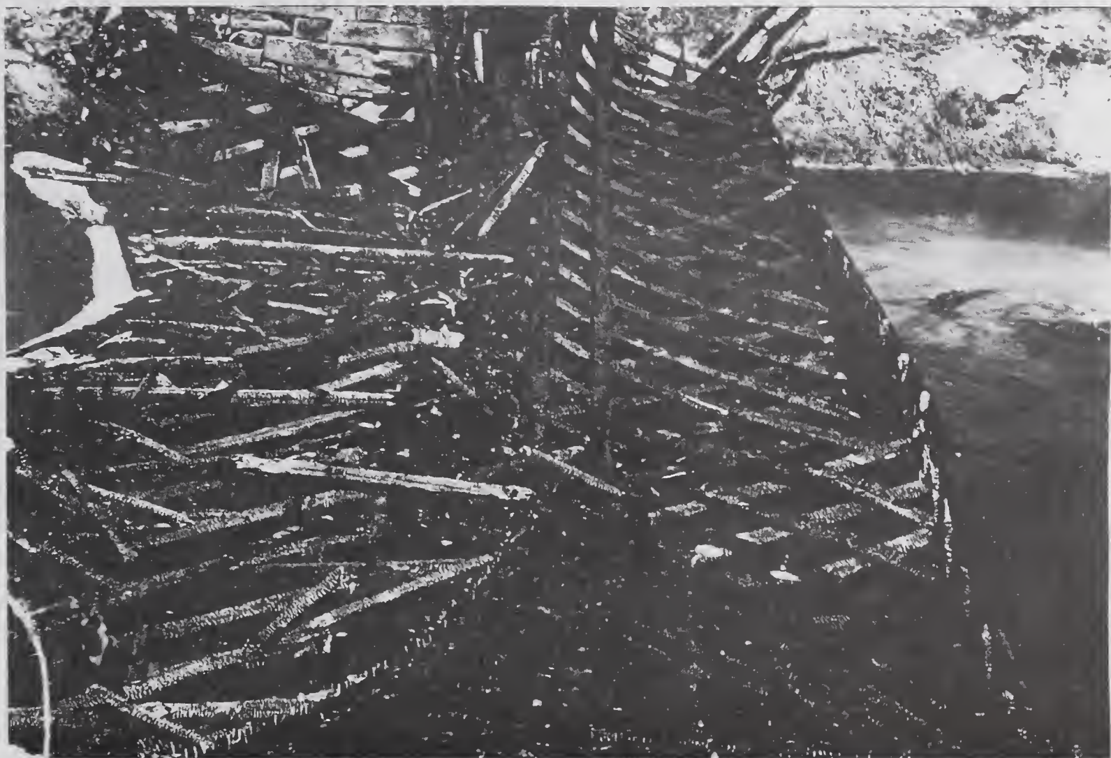
Merrimack was fortunate to have two covered bridges. Both the Turkey Hill Bridge and Field's Bridge spanned the Merrimack River. Within one year, in the 1960's, both were destroyed by arsonists.
