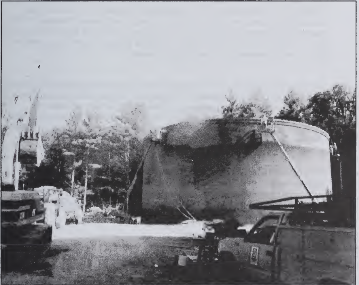
Water Tank Project - Summer St. Bob Naylor Photo
