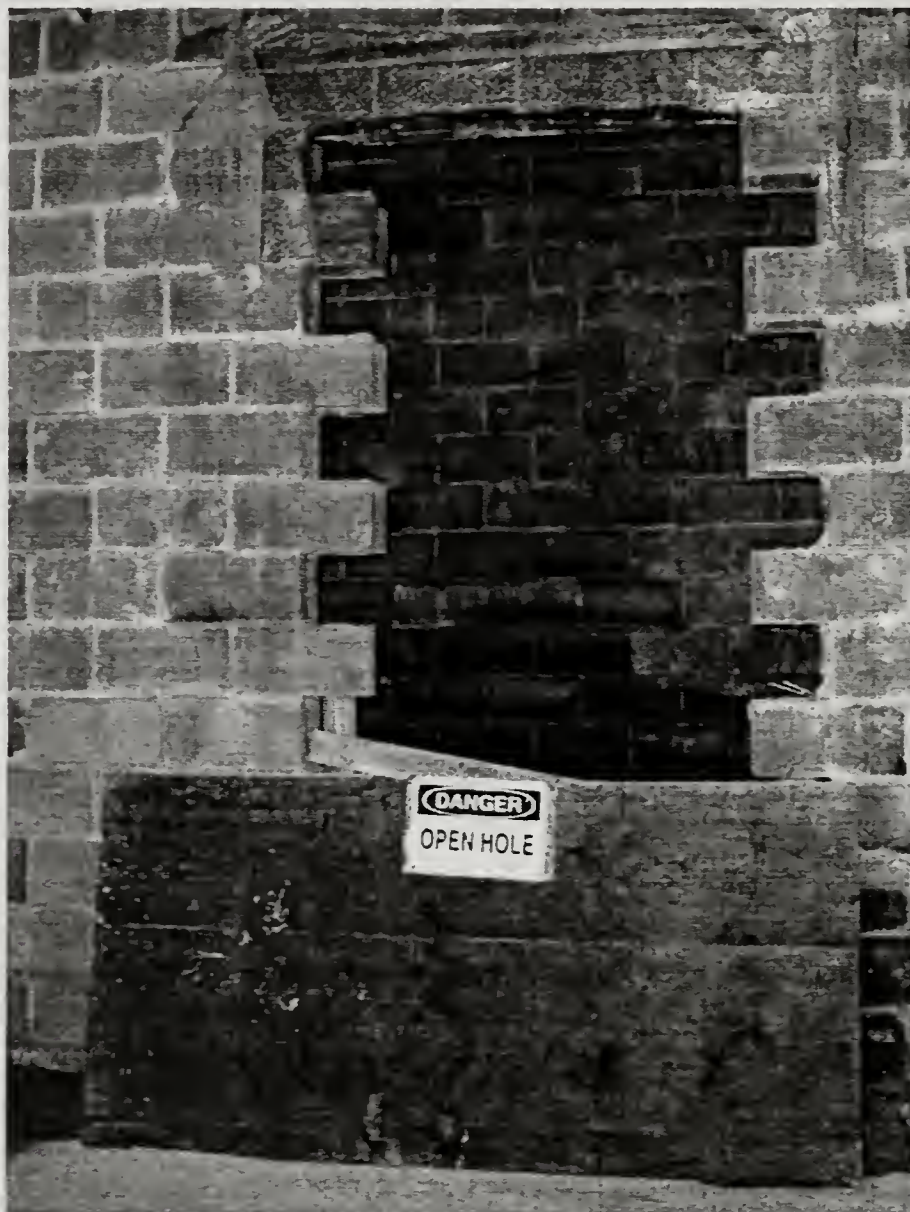
Construction on the new middle school
