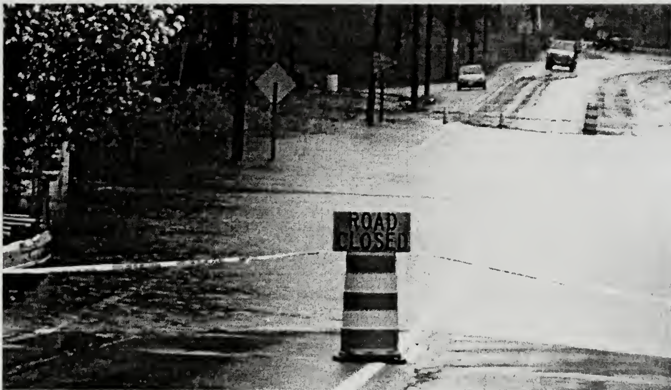
Route 27 during the flood.
